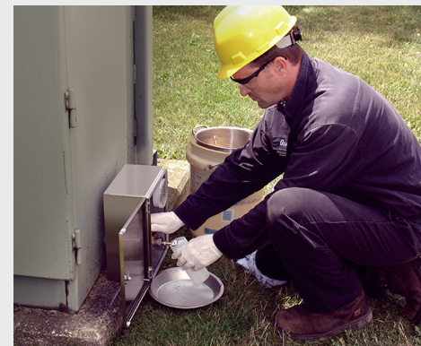
External Oil Sampling – Courtesy of SDMyers
